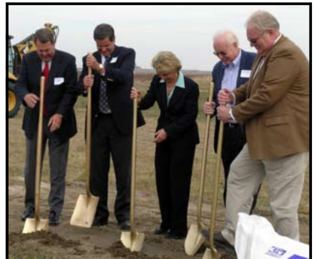
Dirt is turned and construction is officially started on Guardians 500,000 square foot facility in Moses Lake
