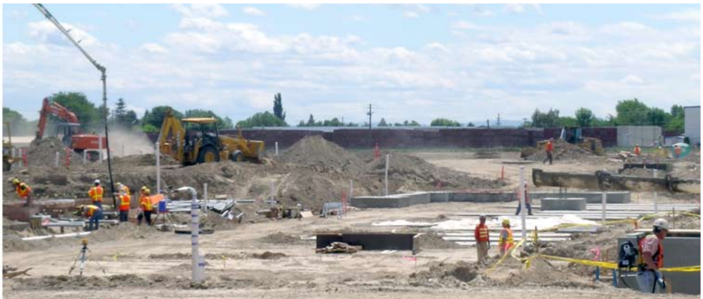
Construction on the Microsoft Data Center as of June 16
