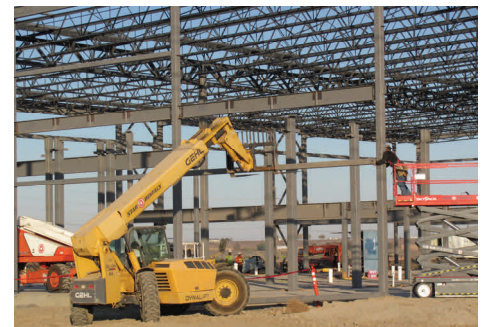
Construction of AstaReal in Moses Lake, October 2013
