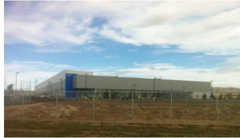
Vantage Data Center, Quincy, WA
